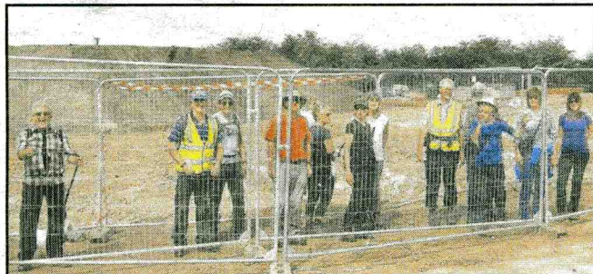
Sandbach Footpath Group fuming by the foundations on the footpath.
